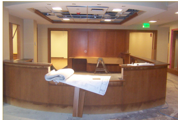
ABOVE: The new library circulation desk under construction in January 2010.
